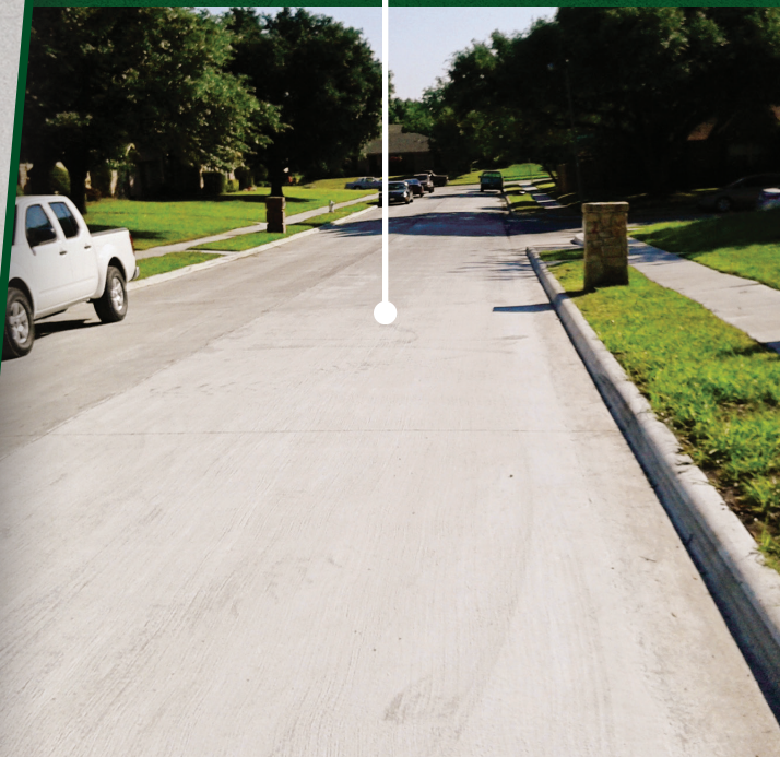
Example of concrete street rated Grade 4 after repair.
