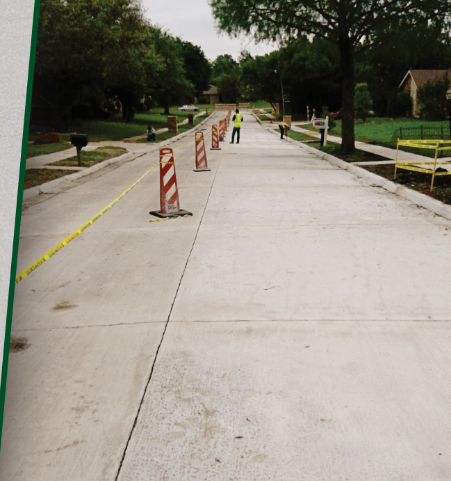
Example of concrete street rated Grade 4 after repair.
