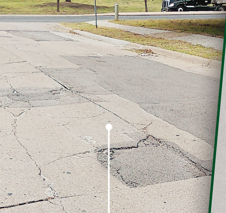
Example of concrete street rated Grade 4 before repair.
