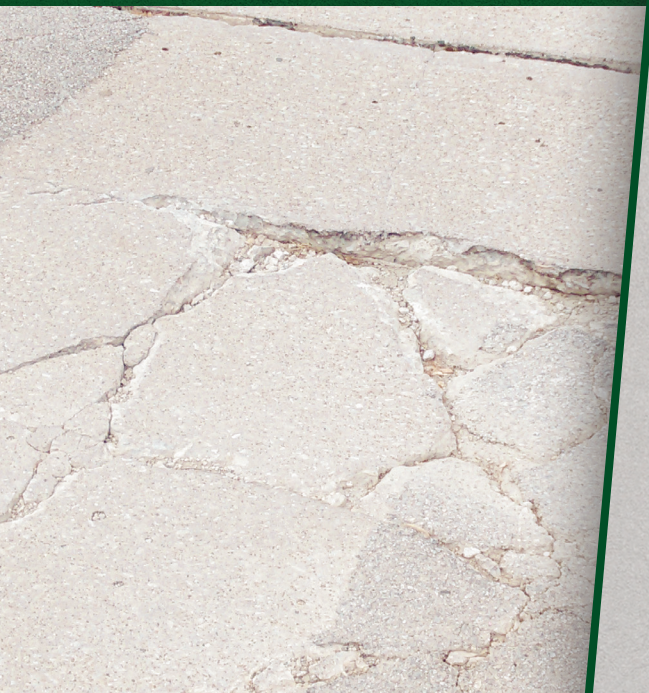
Example of concrete street rated Grade 4 before repair.
