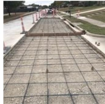
**What's happening now and work expected in the next 30 days:** Street repair is progressing through the Indian Trails Subdivision. The contractor is working on the last street in this neighborhood, Osage Trail. All other streets are finished with concrete work and are undergoing clean-up and sod work. Visit [www.cityofmesquite.com/RealTexasRoads/IndianTrails](http://www.cityofmesquite.com/RealTexasRoads/IndianTrails) for details and updates.
