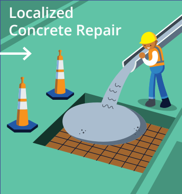
Localized Concrete Repair Small areas of concrete street, sidewalk and curb are cut out and replaced.
