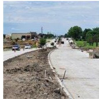
**What's happening now and work expected in the next 30 days:** Retaining walls are being built to provide extra support, while work continues on the trail and medians on Gus Thomasson Road. The new pavement markings are being painted on the road, then all lanes will reopen, and traffic will return to normal.
