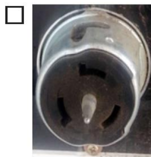
120/240 Volt, 50 Amps, Twist Lock – 3 Wire
