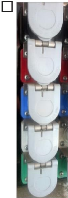
100 Amps, Cam or Cannon plug
