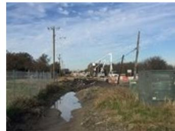
**What's happening now:** All waterlines are complete and passed. Scyene Road pavement is in place from Clay Mathis to the entrance of Ashley Furniture. Franchise utilities are being relocated for pavement to be placed.
