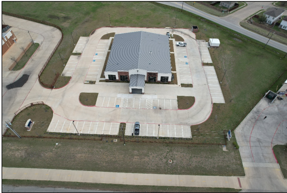
Aerial view (Military Parkway) of subject property
