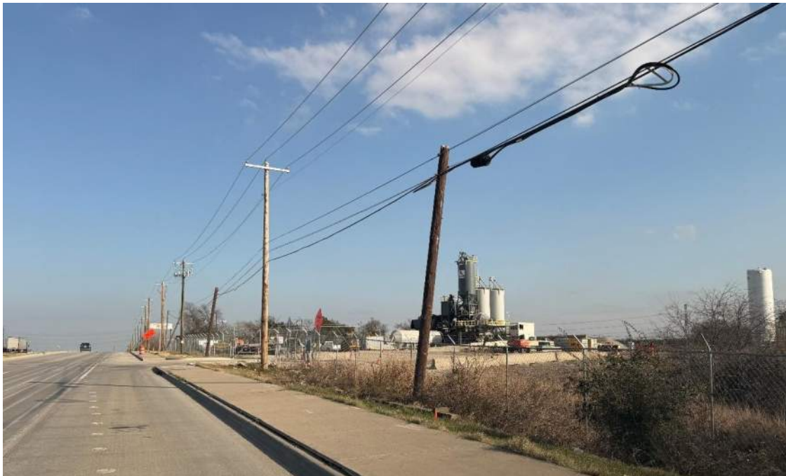
Temporary Batch Plant
