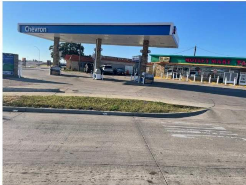
Figure 1 - 2101 Motley Drive - Chevron Gas Station
